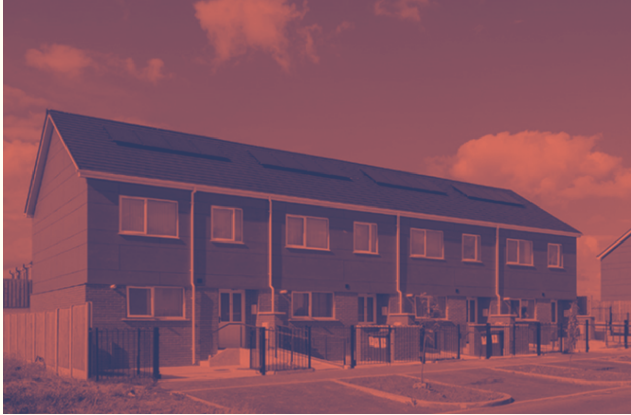
Figure 2. Ballymun Rapid Build exterior
